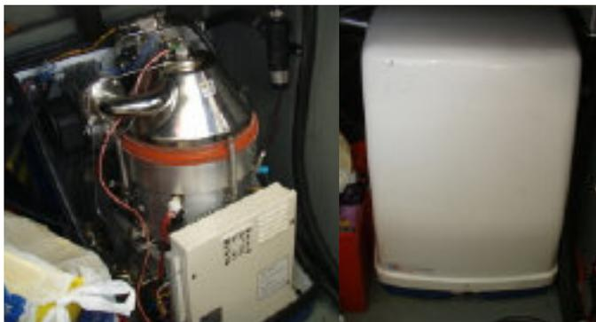
The DC WhisperGen™ heat and power system is a uniquely quiet, independent power generation and heating system adapted for the marine sector, mobile, and remote home environments. It provides power to automatically charge batteries that run all of the onboard / remote applications anytime. It automatically provides hot water and also heat for a warm and dry living environment inside.
